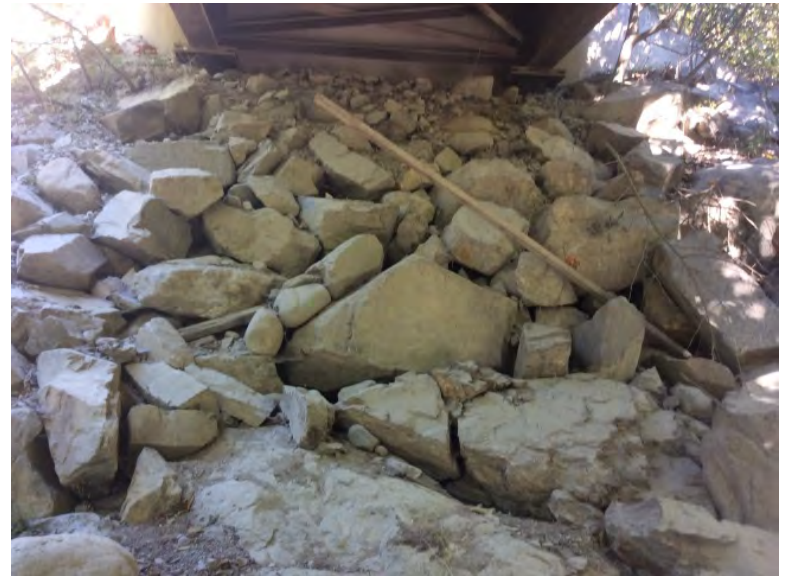
Right Bank Abutment when facing downstream
