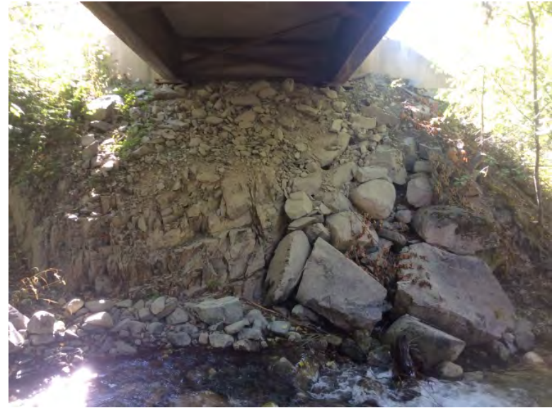
Left Bank Abutment when facing downstream
